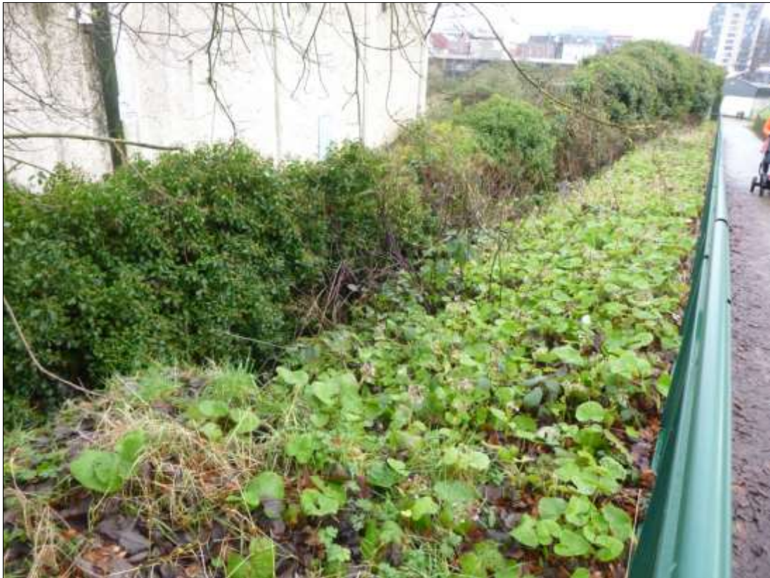
FEBRUARY 2021 – ZONE OF INFESTATION LOOKING SOUTH EAST
